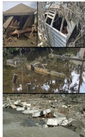
Fig. 2. Typical examples of destroyed timber buildings (top and middle) and destroyed RC with masonry infill structure (bottom).
